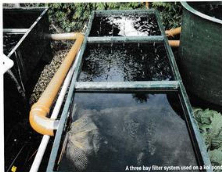
A three bay filter system used on a koi pond
